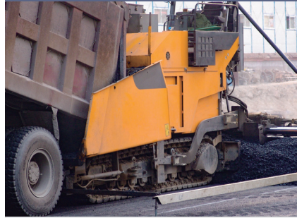
筑路机械 Road Construction
